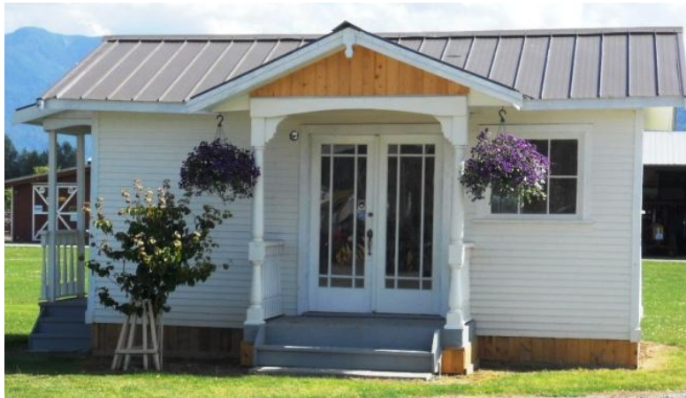
Exterior almost complete
